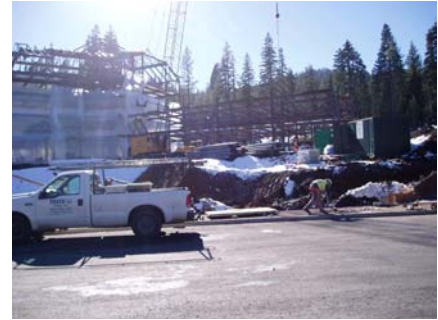
Section of Building J not yet weatherproofed.
