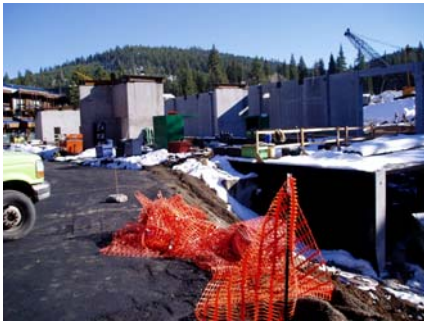
Building H takes on it's first snow.
