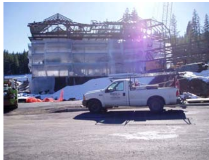
Weatherproofing going up in Building J.
